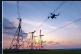
Türkiye: Power transmission line inspection
